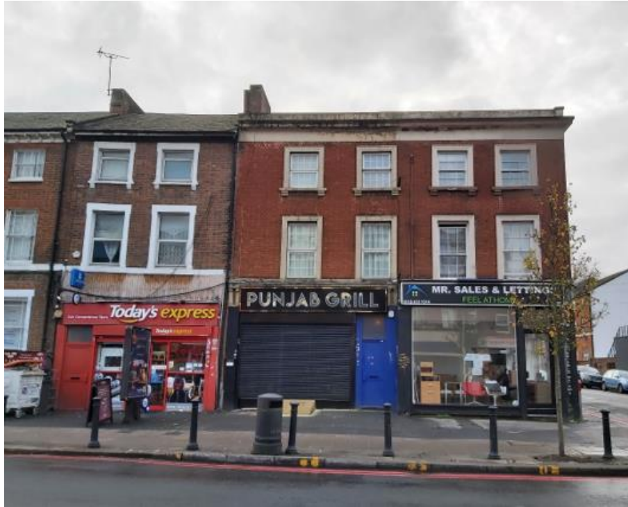
Photo of application site on the corner from 2020.
